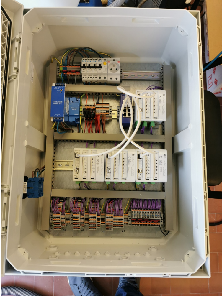
1166 Figure A7. Electrical cabinet used for SalTExPreS
