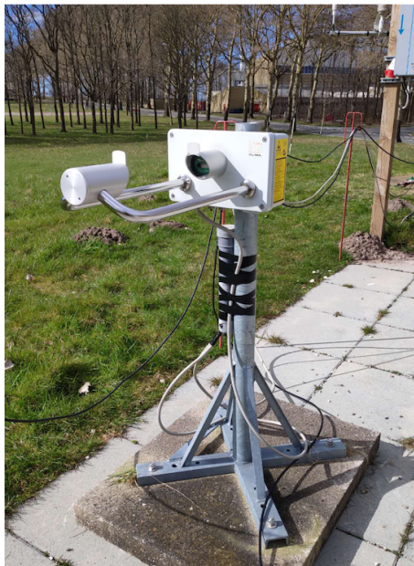
Figure 5. Thies Laser Precipitation Monitor (LPM) at DTU Risø campus.
