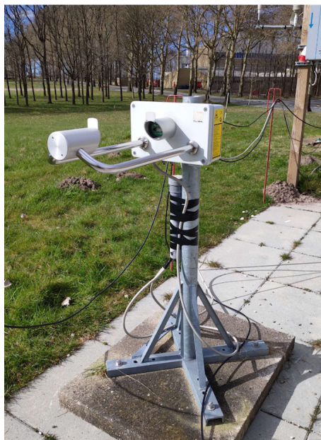
Figure 6: Thies Laser Precipitation Monitor(LPM) at DTU Risø campus.
