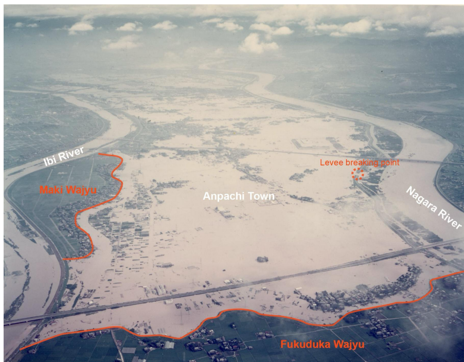
305 Figure 5: September 1976 flooding. The Nagara River levee broke, and the floodwaters flowed out onto the floodplain, where Anpachi town was located. However, the floodwaters were prevented from expanding into the inundated area by the remaining ring levees (courtesy of the Ministry of Land, Infrastructure, Transport and Tourism).
