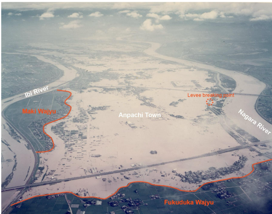
310 Figure 5: September 1976 flooding. The red lines in the photo indicate remaining ring levees. The Nagara River levee broke, and the floodwaters flowed out onto the floodplain, where Anpachi town was located. However, the floodwaters were prevented from expanding into the inundated area by the remaining ring levees (courtesy of the Ministry of Land, Infrastructure, Transport and Tourism).
