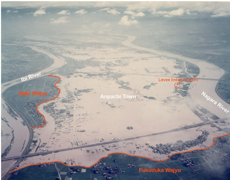
Figure 5: September 1976 flooding. The red lines in the photo indicate remaining ring levees. The Nagara River levee broke, and the floodwaters flowed out onto the floodplain, where Anpachi town was located. However, the floodwaters were prevented from expanding into the inundated area by the remaining ring levees (courtesy of the Ministry of Land, Infrastructure, Transport and Tourism).
