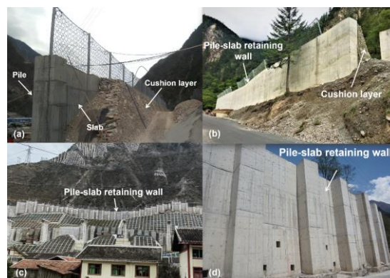
79 80 Fig. 1. PSRW in south-western China (a) Kongyu town (b) Jiuzhaigou nature reserve (c) Zhenjiangguan 81 tunnel exit in Chengdu-lanzhou railway (d) Zhangmu town
