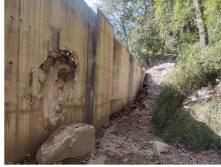
(f) 9m height broken PSRW with no cushion at Zhangmu port in Tibet
