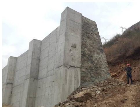
(d) 5m height PSRW with sand cushion at Kangding county
