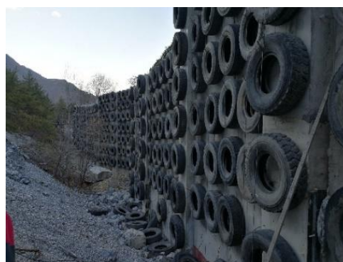
(b) 4 m height PSRW with tyre cushion at Kangding county
