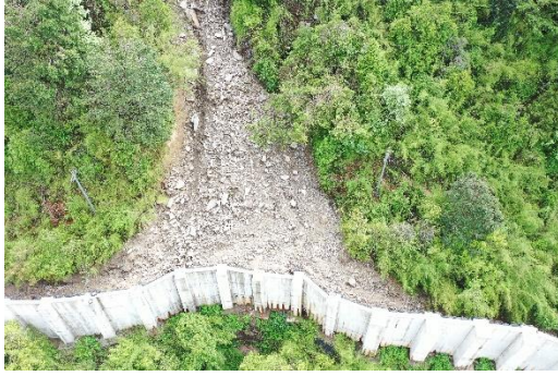
(e) 9m height PSRW with stone cushion at Zhangmu port in Tibet
