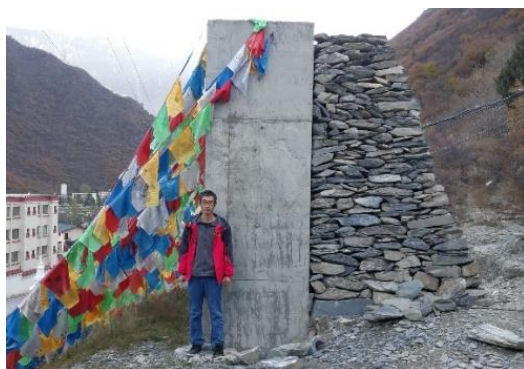
(c) 4m height PSRW with stone cushion at Kangding county
