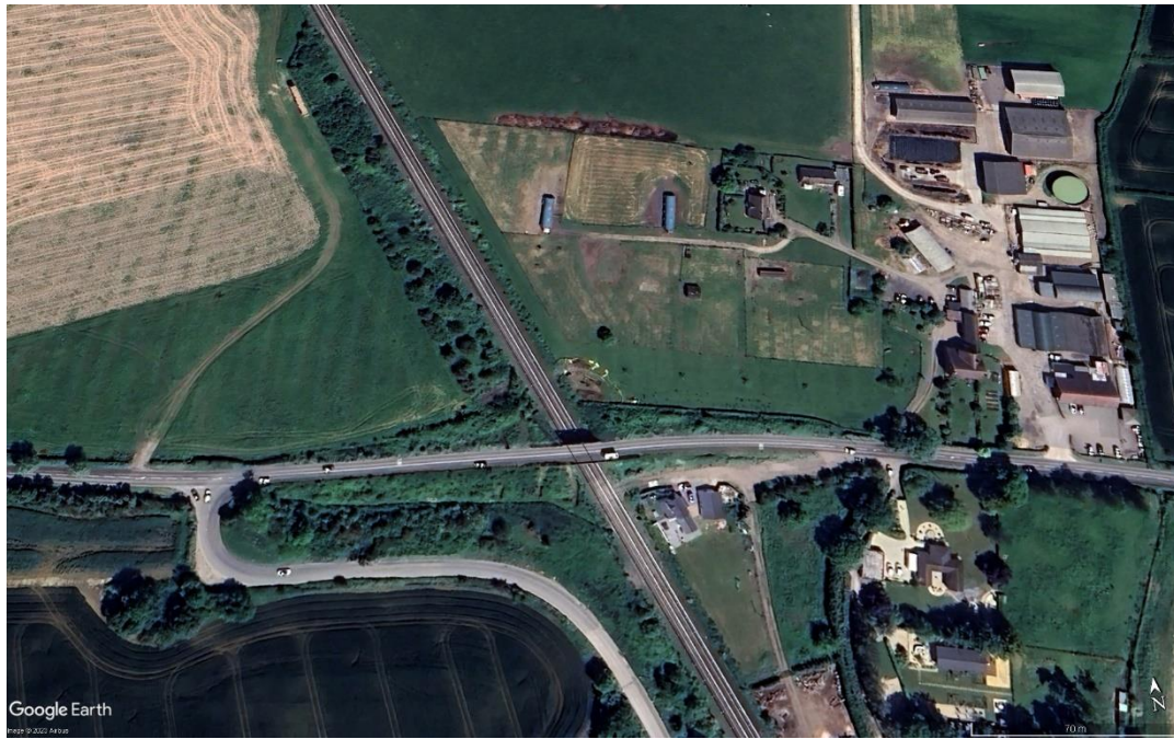
Figure S3. Google Earth Image (Airbus 2023) of the gas leak site taken in June 2023 (Google and Airbus, 2023), showing works being done on the west site of the railway line.
