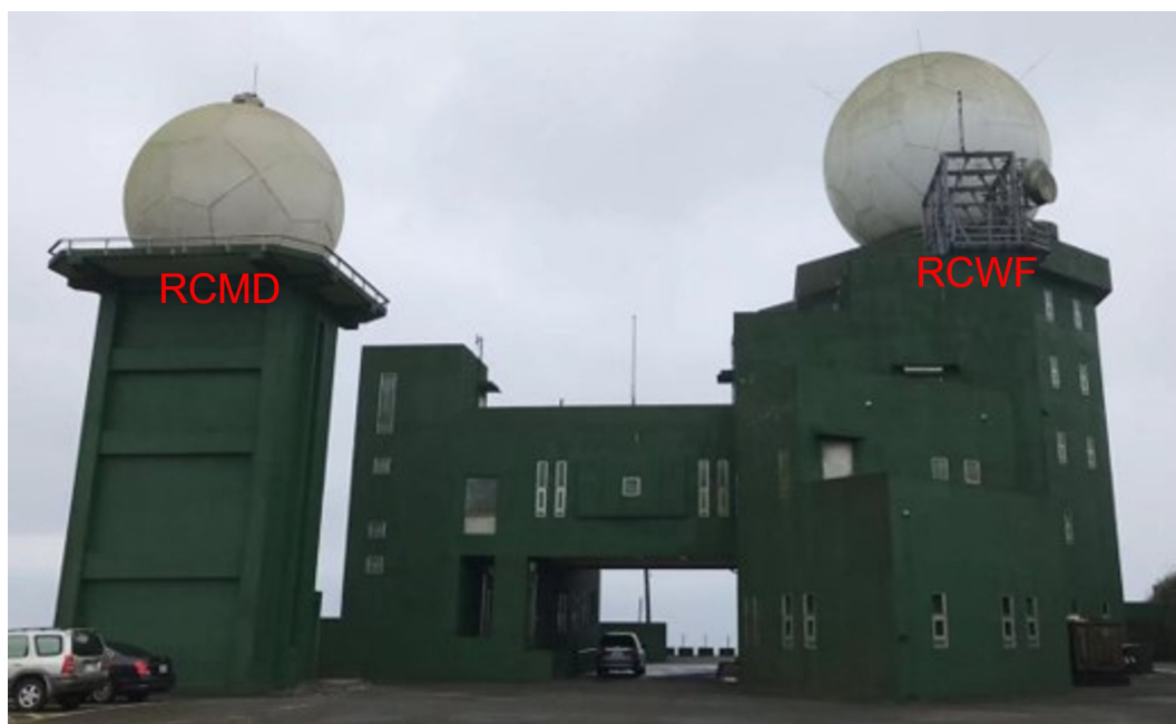
Figure 1. RCMD (C-Band) left and RCWF (S-Band) right at the Wufenshan weather station
