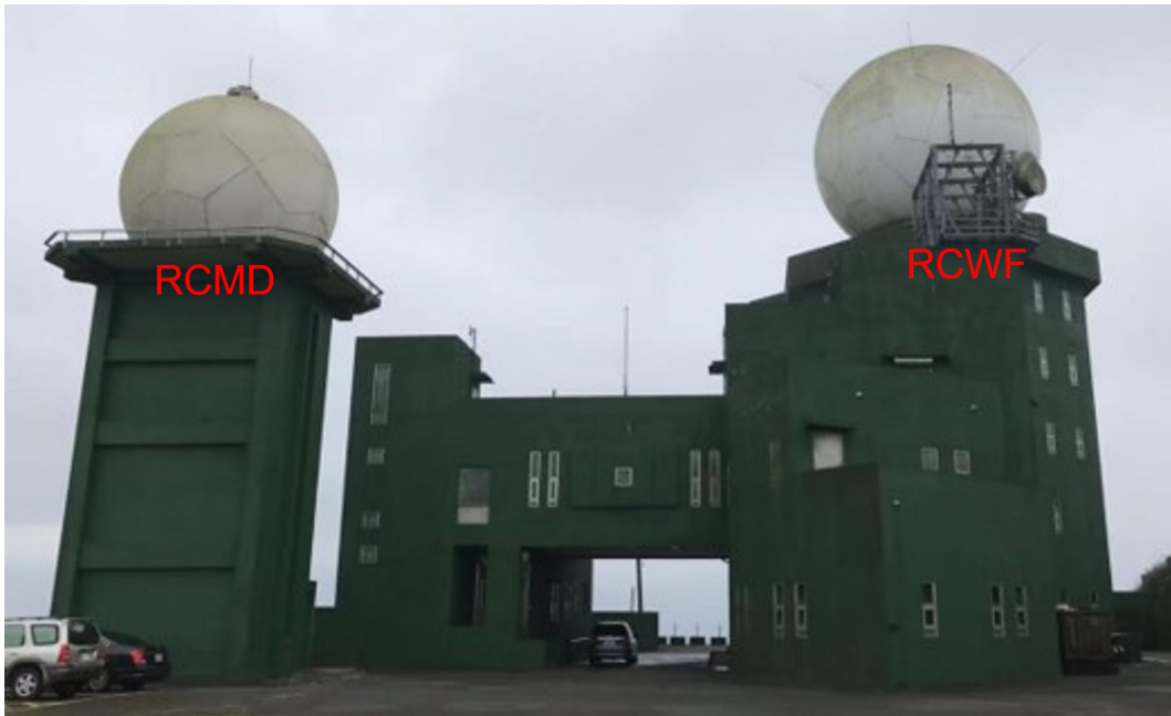
Figure 1. RCMD ( C-Band C-band ) left and RCWF ( S-Band S-band ) right at the Wufenshan weather station
