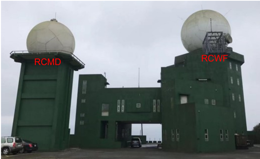
Figure 1. RCMD (C-Band) left and RCWF (S-Band) right at the Wufenshan weather station
