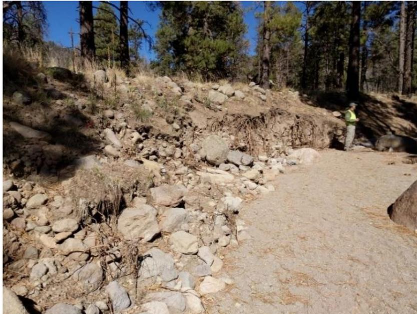
175 **Figure 2. Surveyors performing a BEHI analysis on a typical channel along Spruce Wash. Photo taken in fall 2021 approximately 500 m upstream of Mount Elden Estates.**
