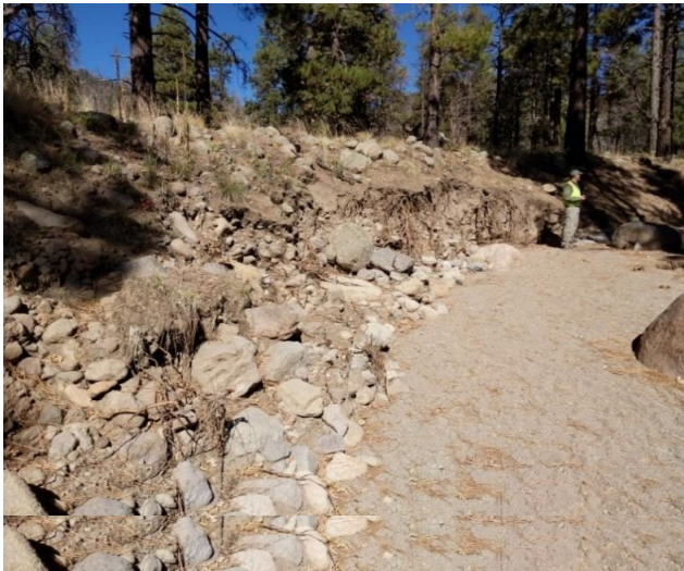
Figure 2. Surveyors performing a BEHI analysis on a typical channel along Spruce Wash. Photo taken in fall 2021 approximately 500 m upstream of Mount Elden Estates.
