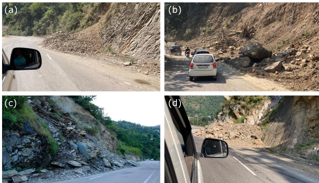
600 Figure 2: Examples of partially road-blocking landslides along the highway NH-7. Panels a) and c) show locations, where hillslopes parallel the foliation/bedding.
