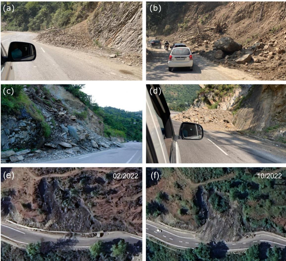
**Figure 2: Examples of partially road-blocking landslides along the highway NH-7.** Panels a) and c) show locations, where hillslopes parallel the foliation/bedding. Panels (e) and (f) show a landslide that was reactivated in the observation period (Google, ©2024 Airbus).
