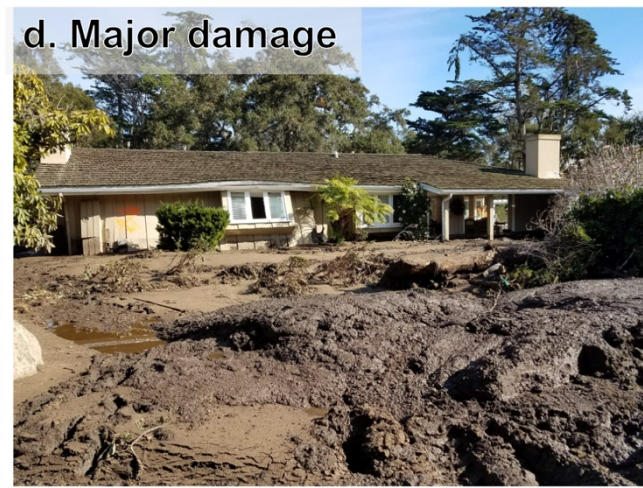
Figure 2. (a,c,d) Examples of buildings that were classified as sustaining major damage or destroyed from different locations in the San Ysidro runout path (locations depicted in Figure 11). Some buildings had the entire first floor wiped out (a, CAL FIRE building damage ID 437), others were inundated by boulders (c, CAL FIRE ID 268), and others were impacted by mud (d, CAL FIRE ID 100). Panel b (CAL FIRE ID 389) depicts a building that had minor damage. All photos from Kean et al. (2019a).
