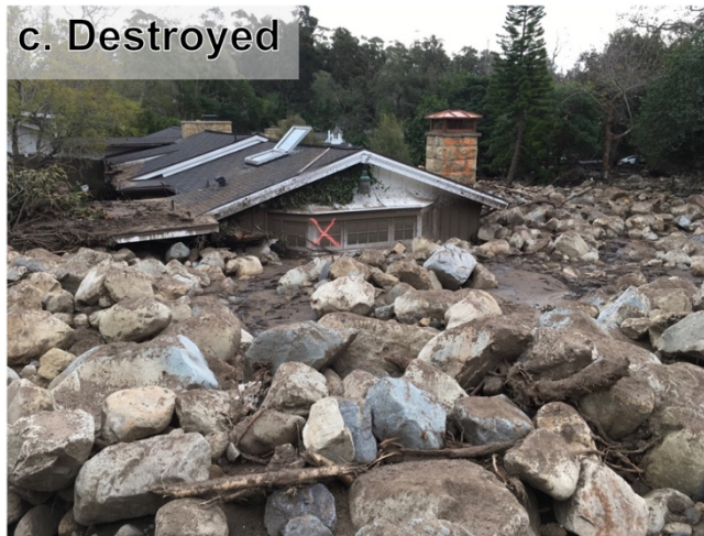
895 Figure 2. (a,c,d) Examples of buildings that were classified as sustaining major damage or destroyed from different locations in the San Ysidro runout path (locations depicted in Figure 11). Some buildings had the entire first floor wiped out (a, CAL FIRE building damage ID 437), others were inundated by boulders (c, CAL FIRE ID 268), and others were impacted by mud (d, CAL FIRE ID 100). Panel b (CAL FIRE ID 389) depicts a building that had minor damage. All photos from Kean et al. (2019a).
