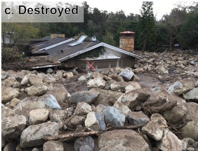
905 | Figure 2. (a,c,d) Examples of buildings that were classified as sustaining major damage or destroyed from different locations in the San Ysidro runout path (locations depicted in Figure 11 Figure 14 ). Some buildings had the entire first floor wiped out (a, CAL FIRE building damage ID 437), others were inundated by boulders (c, CAL FIRE ID 268), and others were impacted by mud (d, CAL FIRE ID 100). Panel b (CAL FIRE ID 389) depicts a building that had minor damage. All photos from Kean et al. (2019a).
