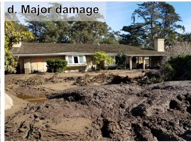
905 | Figure 2. (a,c,d) Examples of buildings that were classified as sustaining major damage or destroyed from different locations in the San Ysidro runout path (locations depicted in Figure 11 Figure 14 ). Some buildings had the entire first floor wiped out (a, CAL FIRE building damage ID 437), others were inundated by boulders (c, CAL FIRE ID 268), and others were impacted by mud (d, CAL FIRE ID 100). Panel b (CAL FIRE ID 389) depicts a building that had minor damage. All photos from Kean et al. (2019a).
