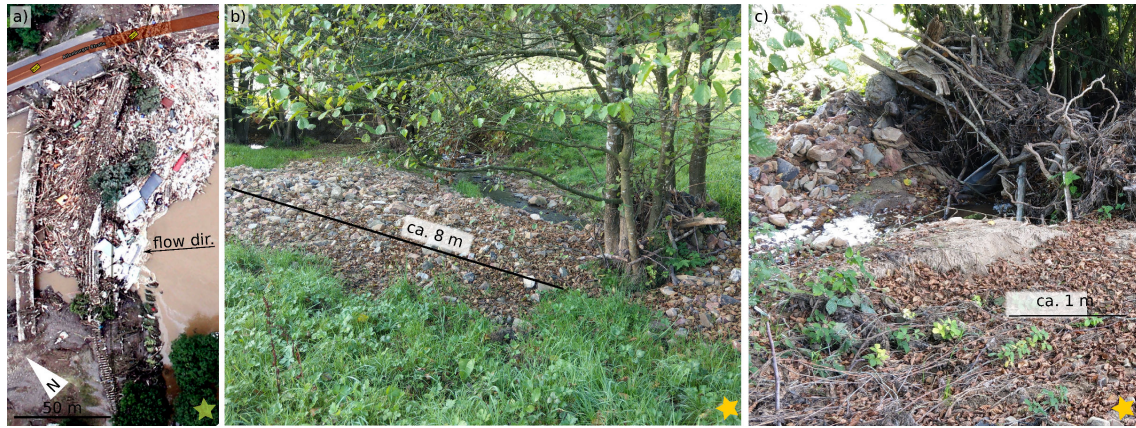
Figure 5. Effects of large woody debris. For locations on wider map see stars in Fig. 1) Pair of clogged bridges near Altenahr, bypassed along the left and right bank. Note the bipartition of the collected debris with woody material caught by the downstream road bridge and anthropogenic debris collected later by the upstream railway bridge. Note two remaining standing trees in the river depicting the width of the Ahr river before the flood. Aerial image by (BBK-DLR, 2022). b) Huhnenbach near Aremberg about 2 km from its source (see Fig. 1). Note clogging by woody debris at riparian trees and the resulting ejection of coarse bed material out of the channel. c) Another clogging of the Huhnenbach some 20 m upstream of (b), with both ejected coarse debris and deposition of fine sediments in front of the obstacle.
