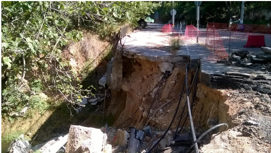
Figure 2: View from the slope failure (fall) of the examined road (Region of Attica/Directorate of Technical Works).
