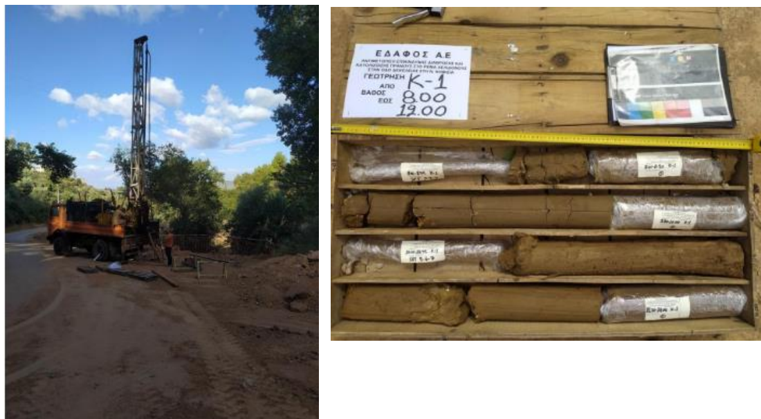
122 Figure 4: Borehole drilling (left photo) and on the right photo a part of the borehole findings (Sand to Clayey geomaterial) 123 from 8.00 – 12.00 meters depth, is depicted (EDAFOS Consulting Engineers, Region of Attica/Directorate of Technical Works).
