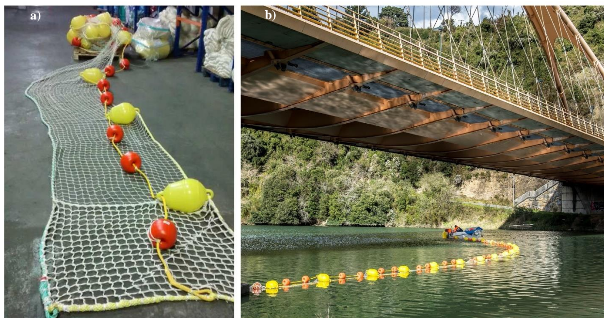
Figure A1. Floating barrier (a) and installation in Deba river (Gipuzkoa) (b)
