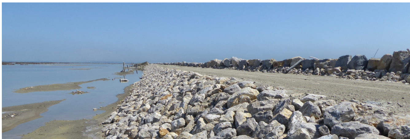
Figure 1. Photo of the landward slope of the dyke
