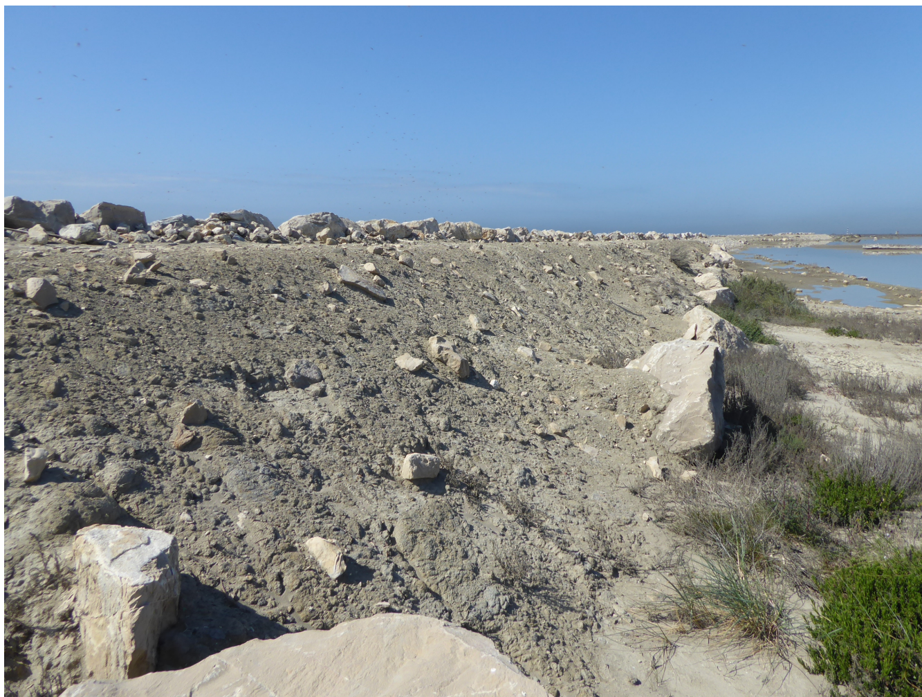
Figure A1. Picture of the landward slope of the dyke
