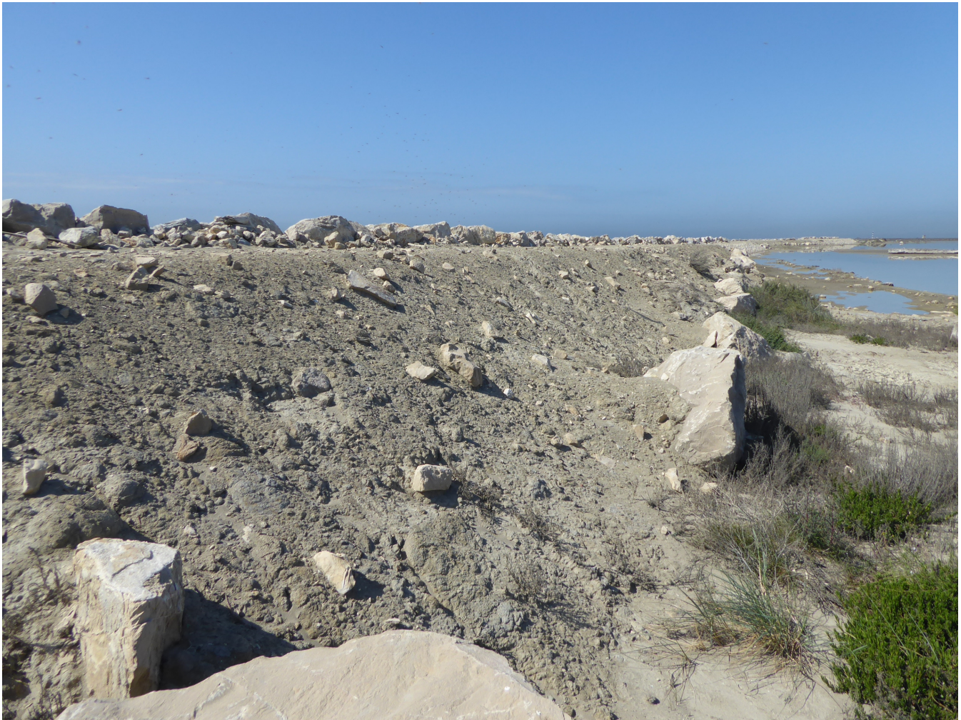
Figure 1. Photo of the landward slope of the dyke
