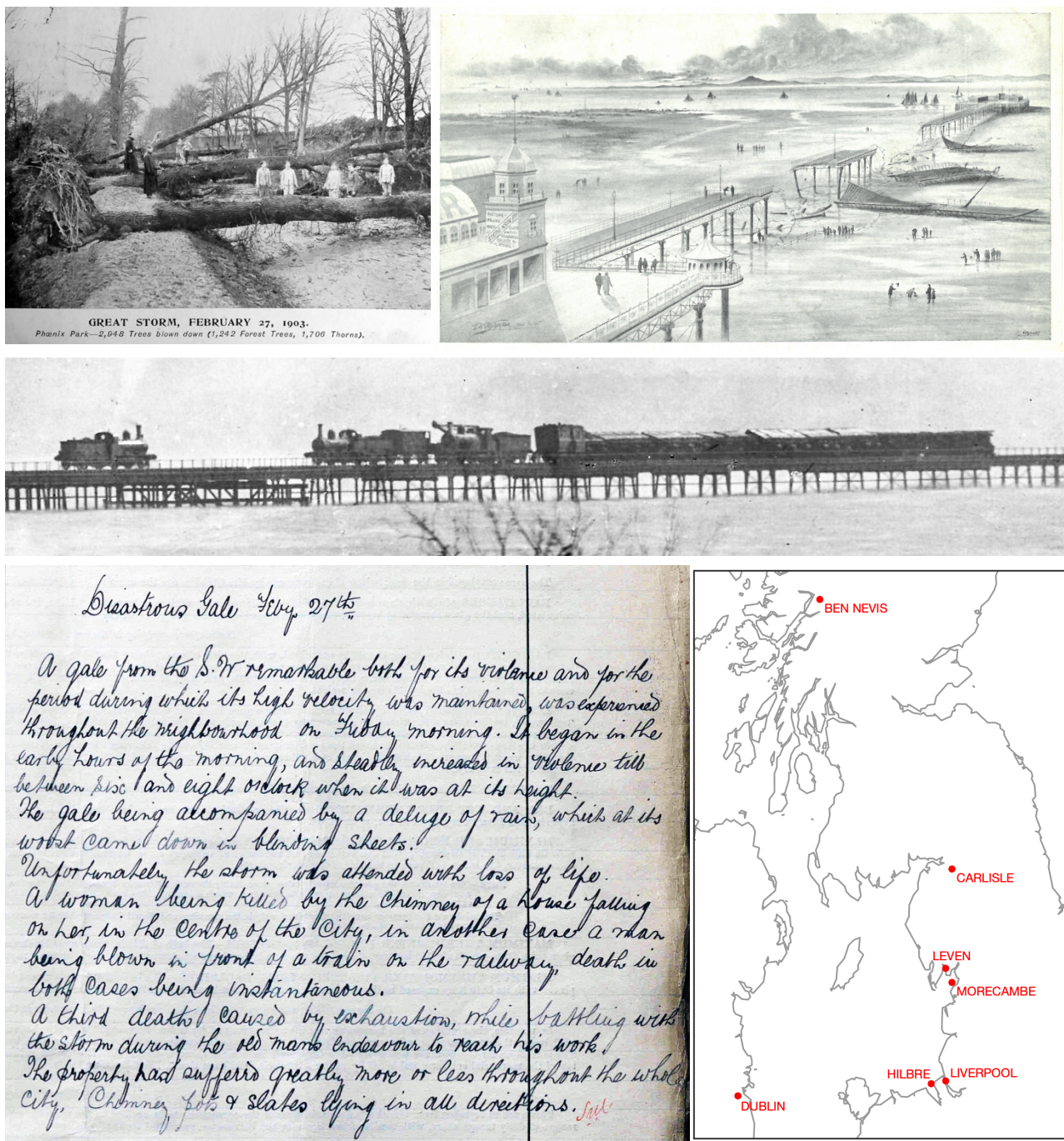
70 Figure 2: Visual descriptions of damage from Storm Ulysses. Top: photographs from Dublin (left) and Morecambe (right). Middle: photograph of a train blown over on Leven viaduct. Bottom: written account of the storm in Carlisle & a map of locations in the photos or named in the text. Dublin image supplied by Aida Yared. The Leven photograph was taken by a Mr Alexander, assistant engineer for the Furness railway. The Morecambe image is a scan of a postcard owned by one of the paper authors.
